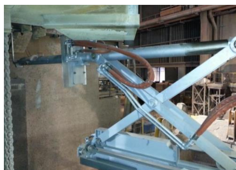
SafEBT-Tap at work, opening the furnace's taphole
