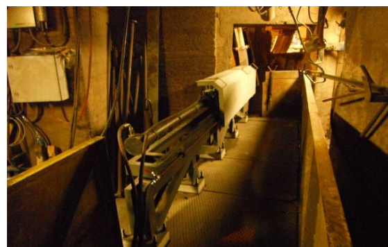
SafEBT-Clean at work, in a dog-house installation
